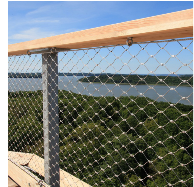
WIRE NET & RAILING CONNECTION EXAMPLE
