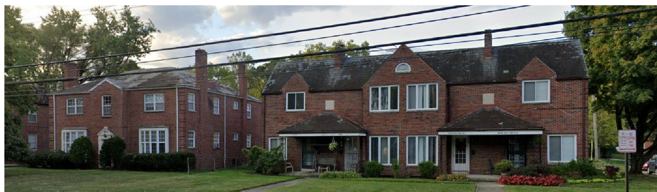
EXISTING MULTIFAMILY BUILDING, EAST LIVINGSTON AT EUCLAIRE AVENUE
