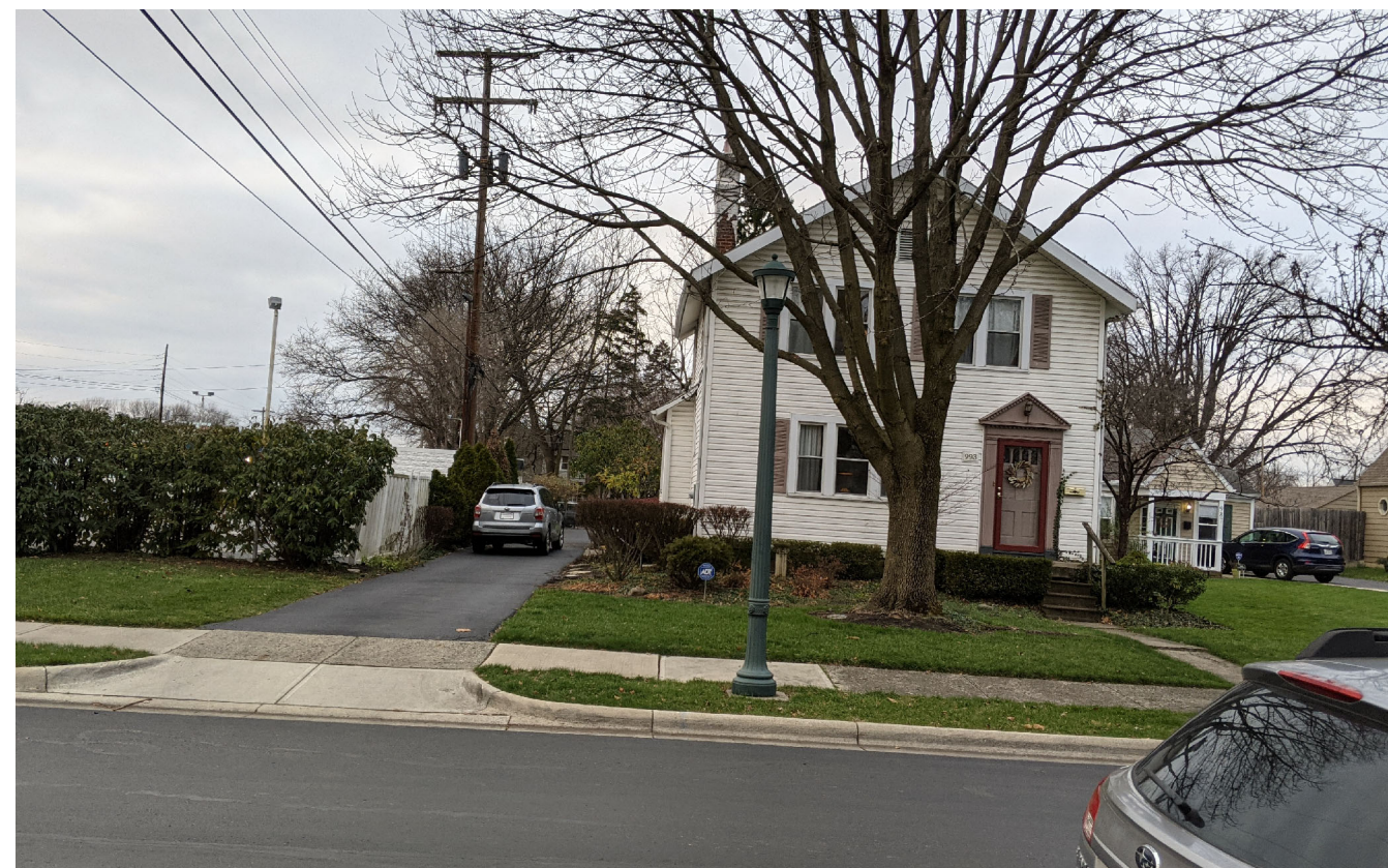
WEST SIDE OF FRANCIS AVENUE
