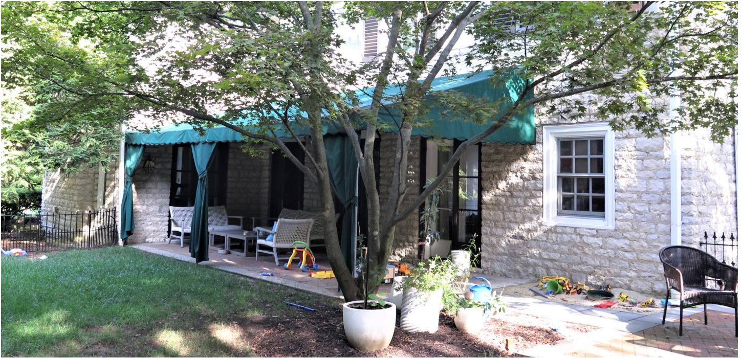
EXISTING SHADE STRUCTURE OVER PATIO
