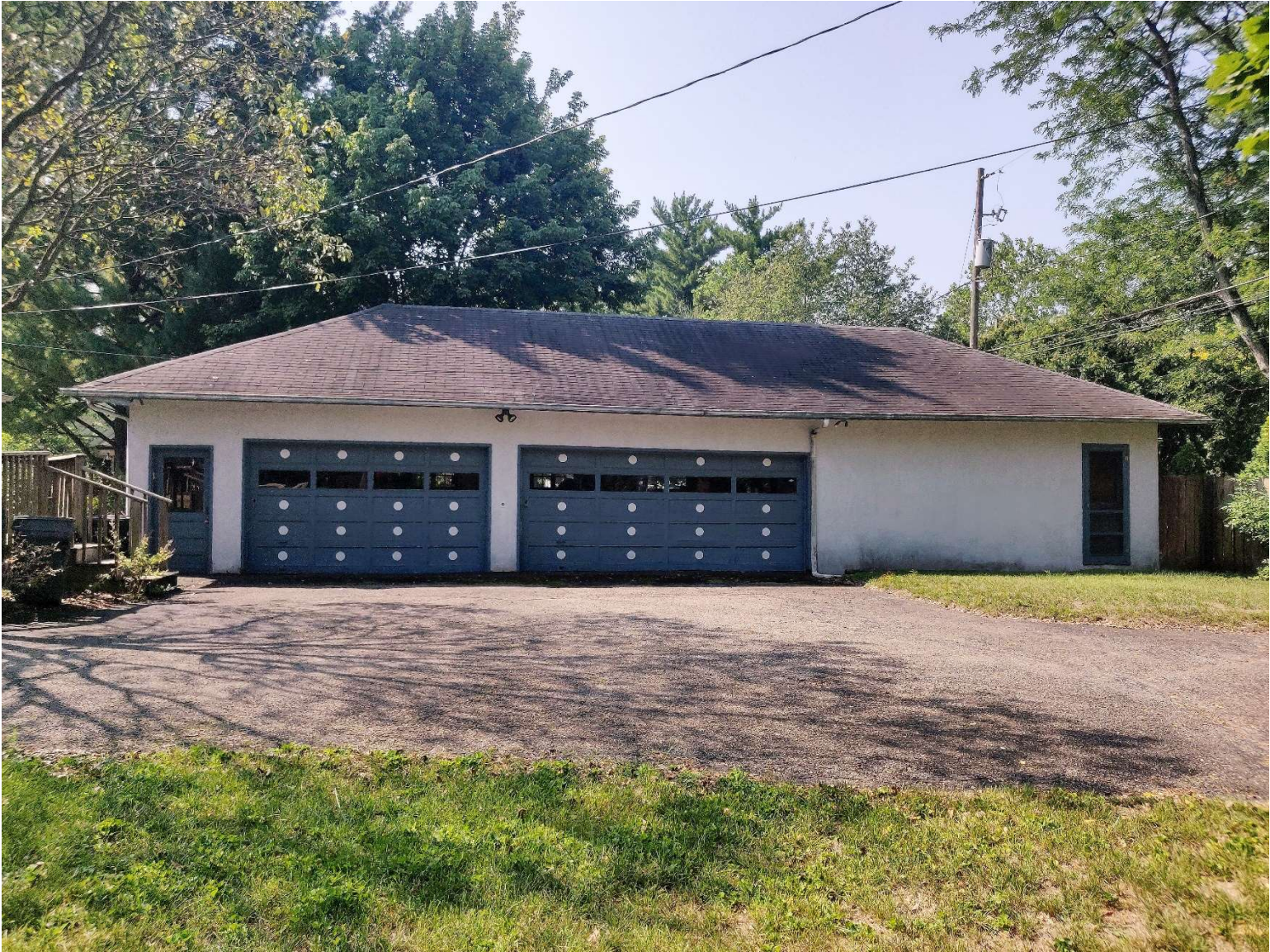
Existing Garage viewed when looking South
