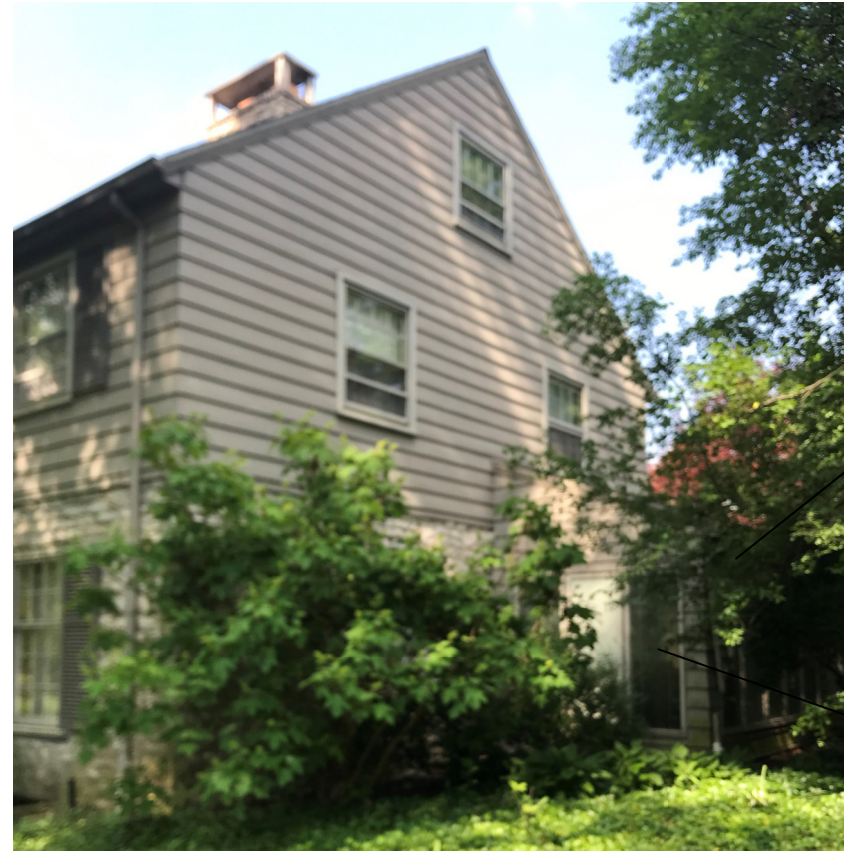
Southwest Corner (Front Right)
