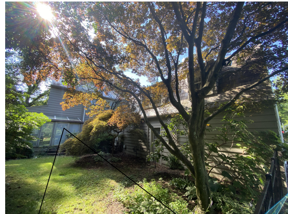
Southeast Corner (Rear Right)
