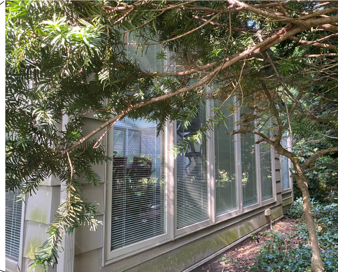
South Wall (Right)
