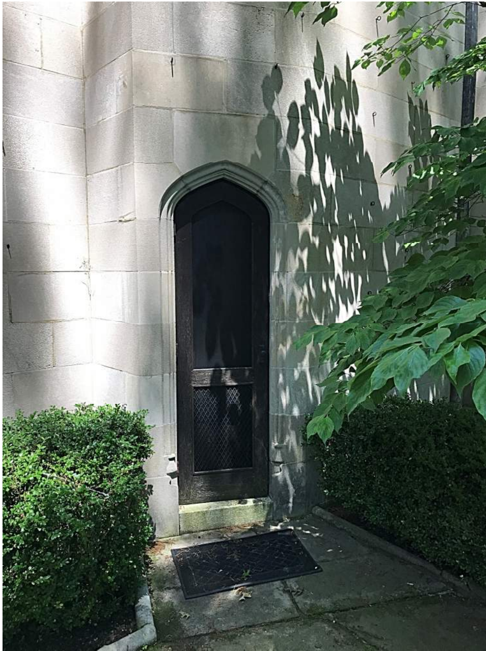
South courtyard, Northeast entry
