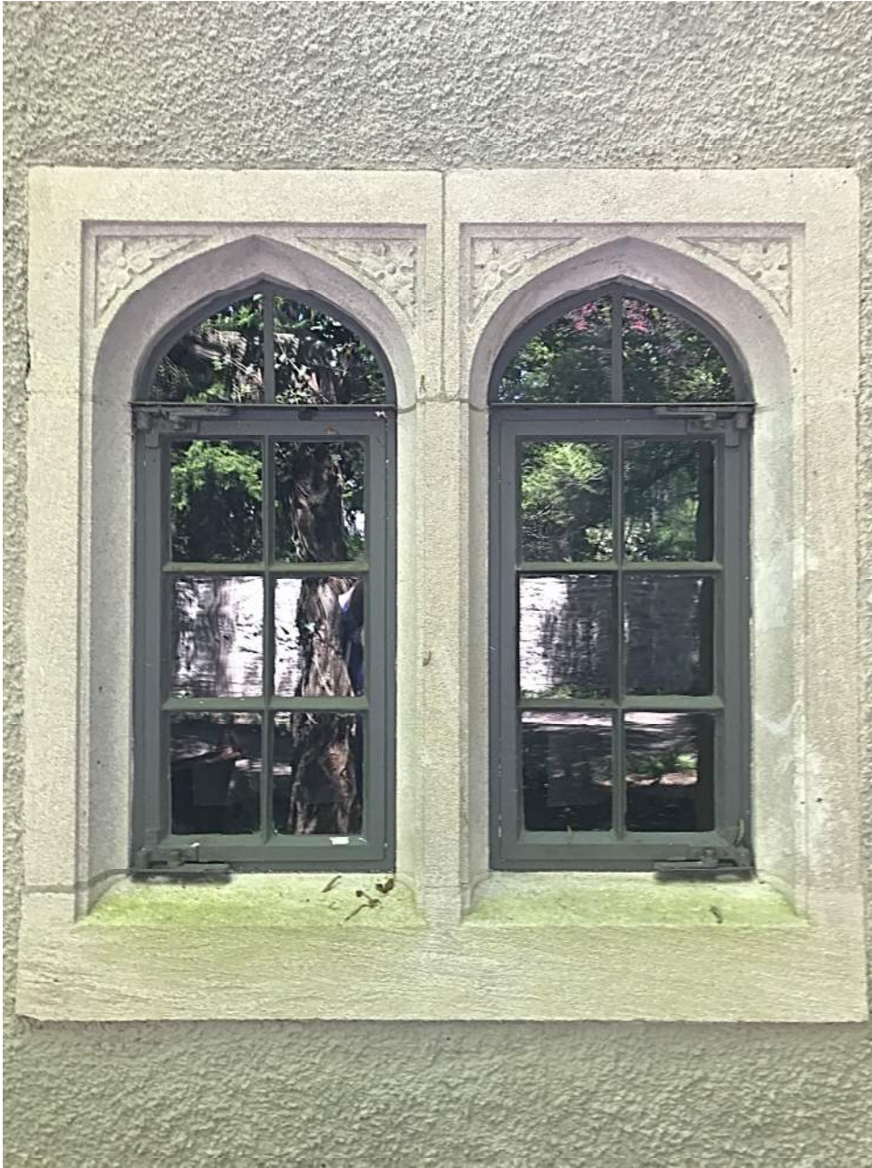
Typical pointed arch top windows
