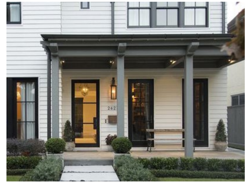
Finish: Timber framing painted gray
