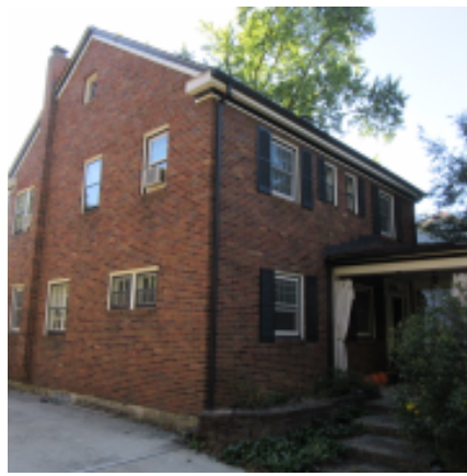
North Elevation Photo Mar 10, 2020
