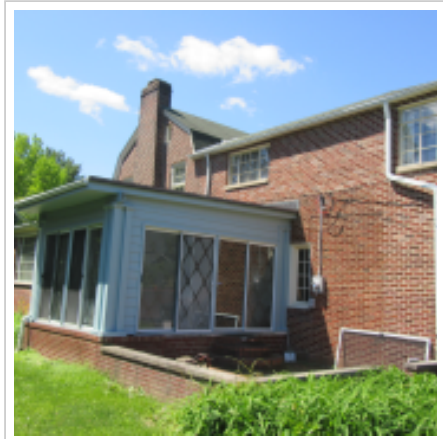
East Elevation Photo II Mar 10, 2020
