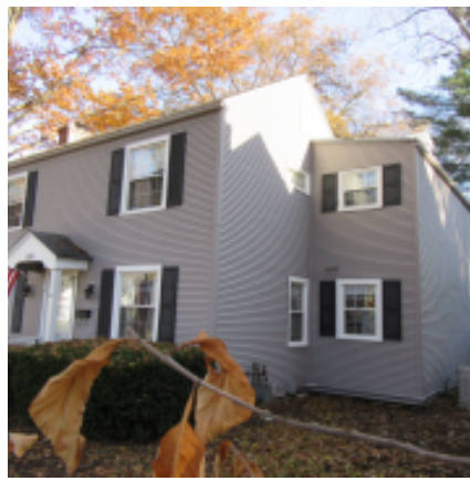
Photo South Elevation Mar 10, 2020
