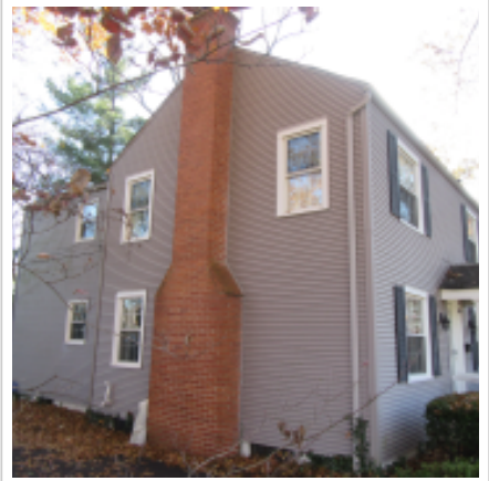
Photo North Elevation Mar 10, 2020
