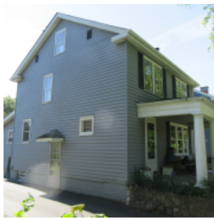
North Elevation Photo Mar 10, 2020
