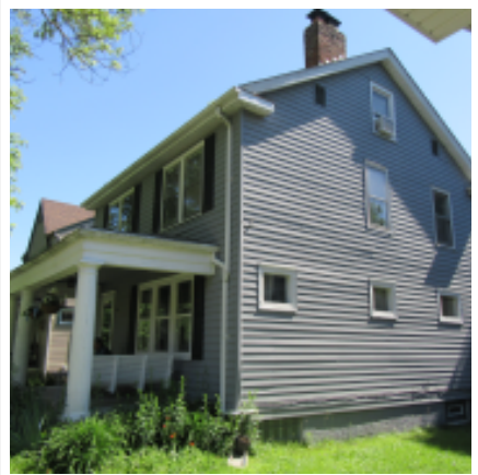
South Elevation Photo Mar 10, 2020
