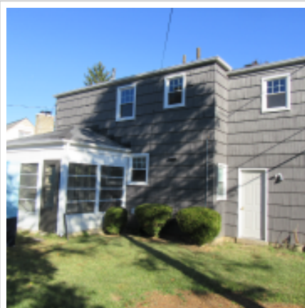
Rear Elevation Mar 10, 2020
