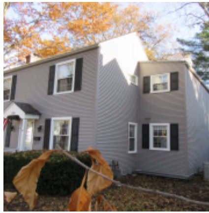
Photo South Elevation Mar 10, 2020
