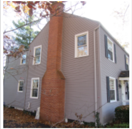
Photo North Elevation Mar 10, 2020
