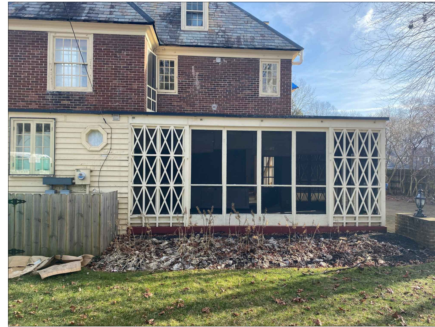
EXISTING PORCH FROM WEST
