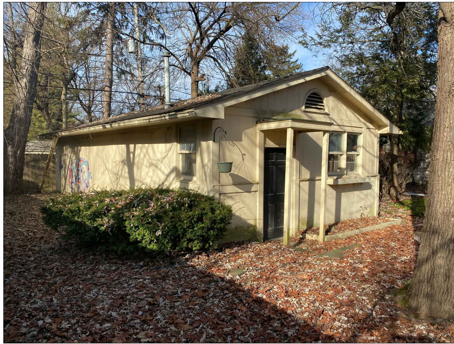
EXISTING GARAGE FROM SOUTHEAST
