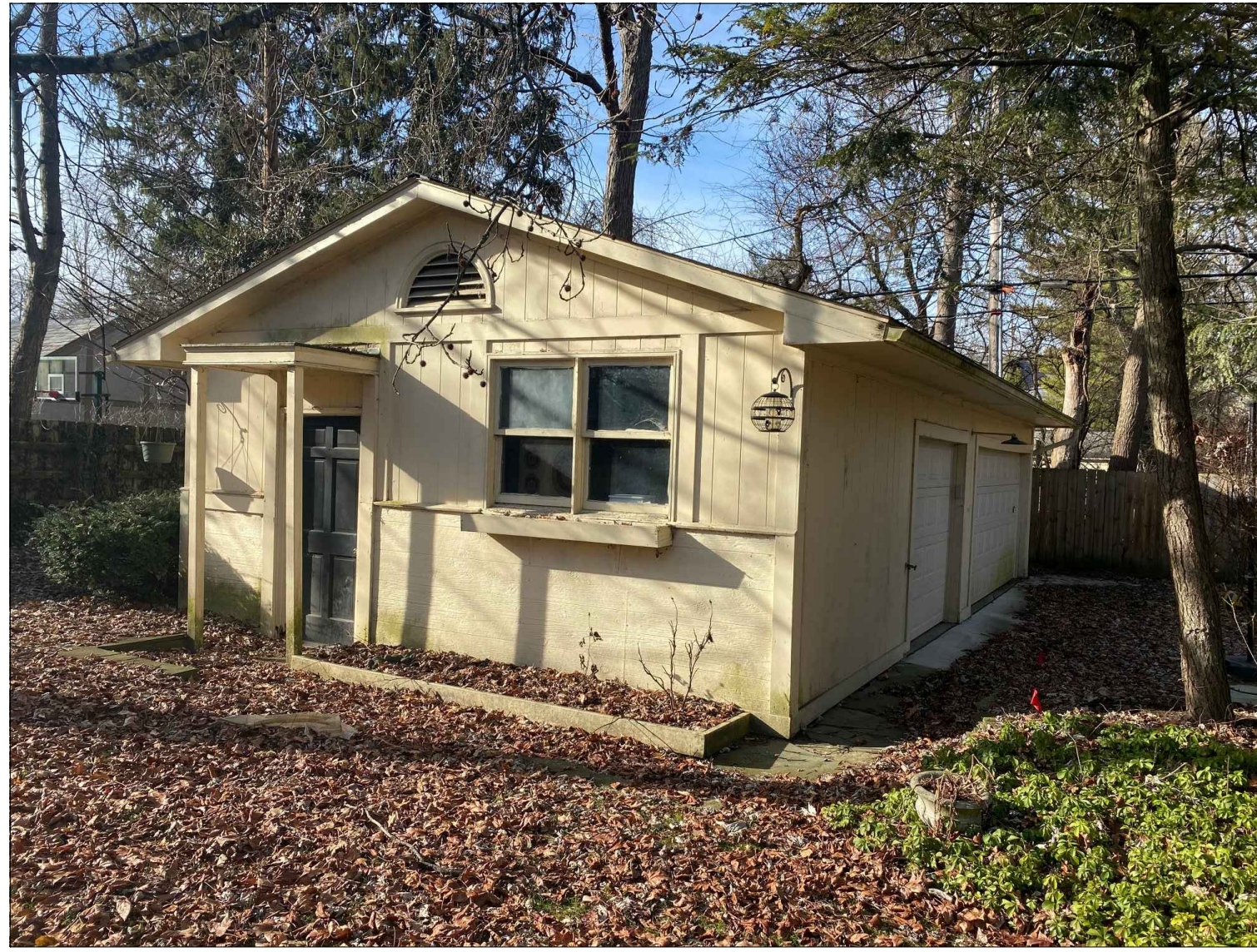
EXISTING GARAGE FROM NORTHEAST
