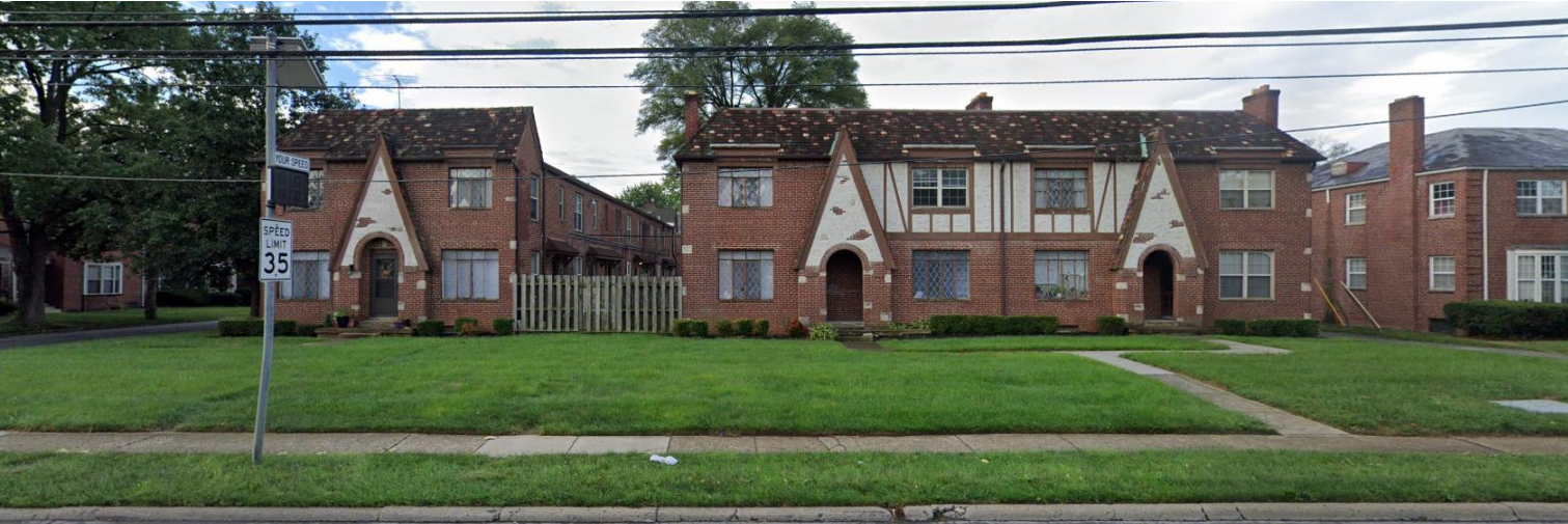
2383-2371 E Livingston Ave (south side of street)
