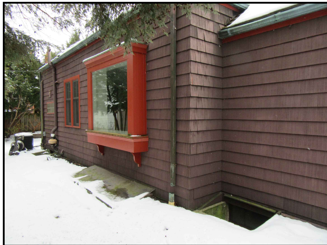
PARTIAL NORTH ELEVATION
