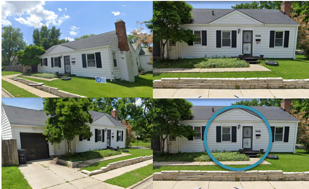
Area of addition
