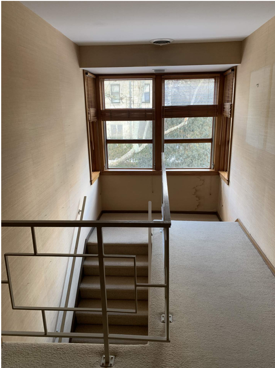
Main Stairwell and Hall
