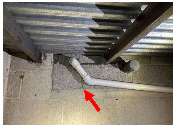
Window well infill and water mitigation framing
