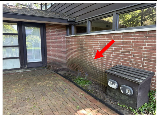
Exterior grade at west side
