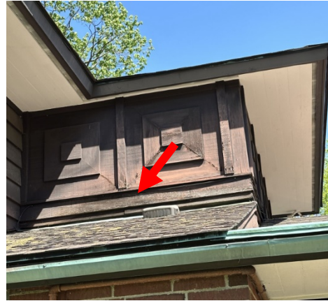
Exterior framing at south low roof
