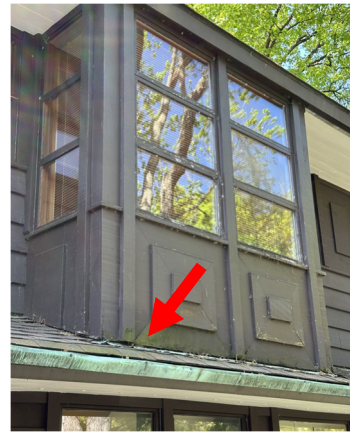
Exterior framing at north low roof
