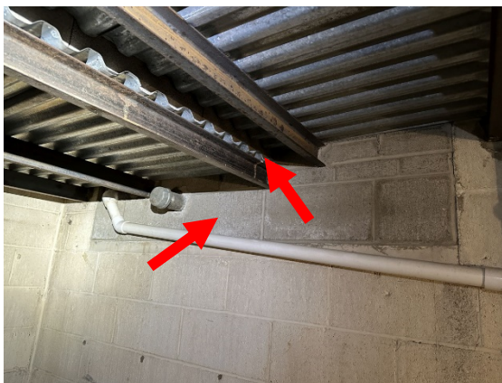
Window well infill and water mitigation framing
