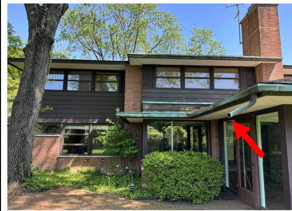
Gutter downspout at south side
