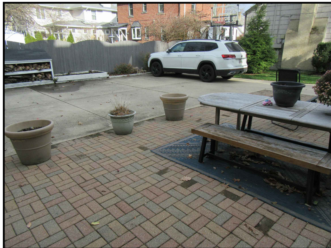
EXISTING PATIO & AUTO COURT LOOKING NORTHEAST
