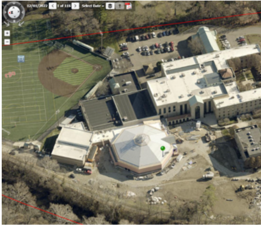
Construction aerial of St. Charles Black roof is the old gym
