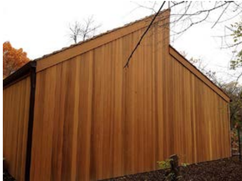
Buffalo Lumber Company A&BTR Clear Cedar milled to 1x6 T&G (V Groove) stained with Olympic 717 "Redwood" Semi-transparent, Oil Based Stain https://www.buffalo-lumber.com/clear-cedar-grade/
