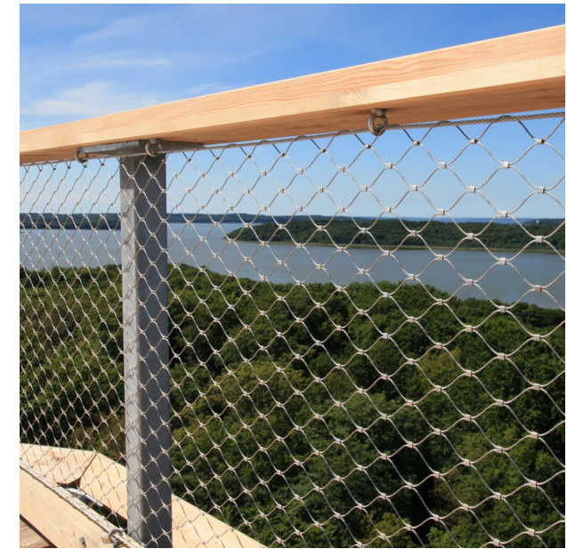
WIRE NET & RAILING CONNECTION EXAMPLE
